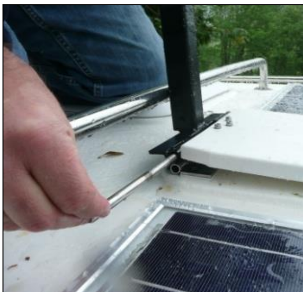
4. Insert Pin Back into Mast
